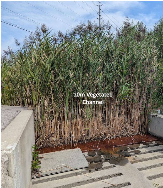
Existing Conditions, Heart Lake SWMF (Region of Peel, in the City of Brampton)
