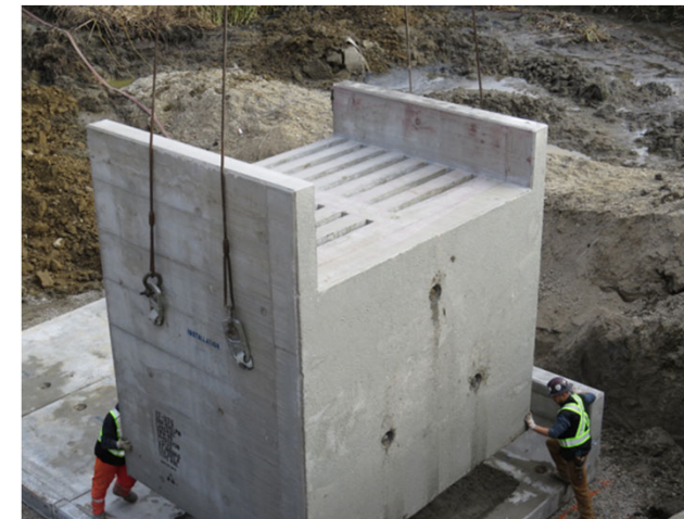
SWM Shield During Construction
