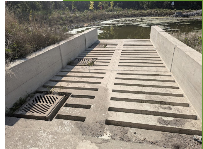
Existing Conditions, Harmonia SWMF, Vaughan
