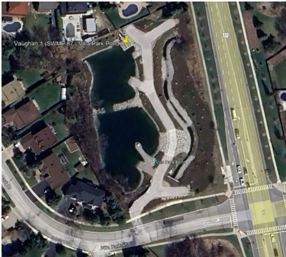
Aerial Image of Villa Park SWMF Pond, Vaughan
