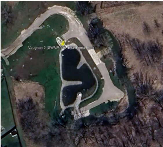
Aerial Image of Harmonia SWMF Pond, Vaughan
